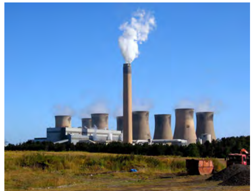
A coal-powered power station.
